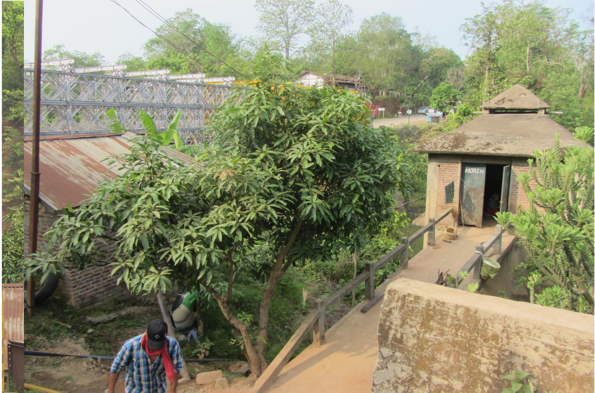
Dry Intake of India side. Pumps are installed at the middle of the intake tower.
